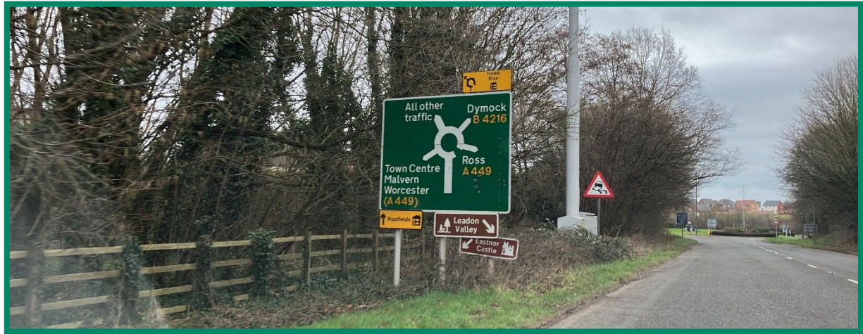
Figure 24 - Existing traffic sign located on the southbound approach to the Leadon Way/ A449 Ross Road roundabout. The sign could be replaced if weight limit introduced on New Street, showing weight limit roundel associated with Town centre. Alternatively a new map type sign showing alternative HGV route and weight limit on New Street is installed on this approach subject to suitable location in verge.
