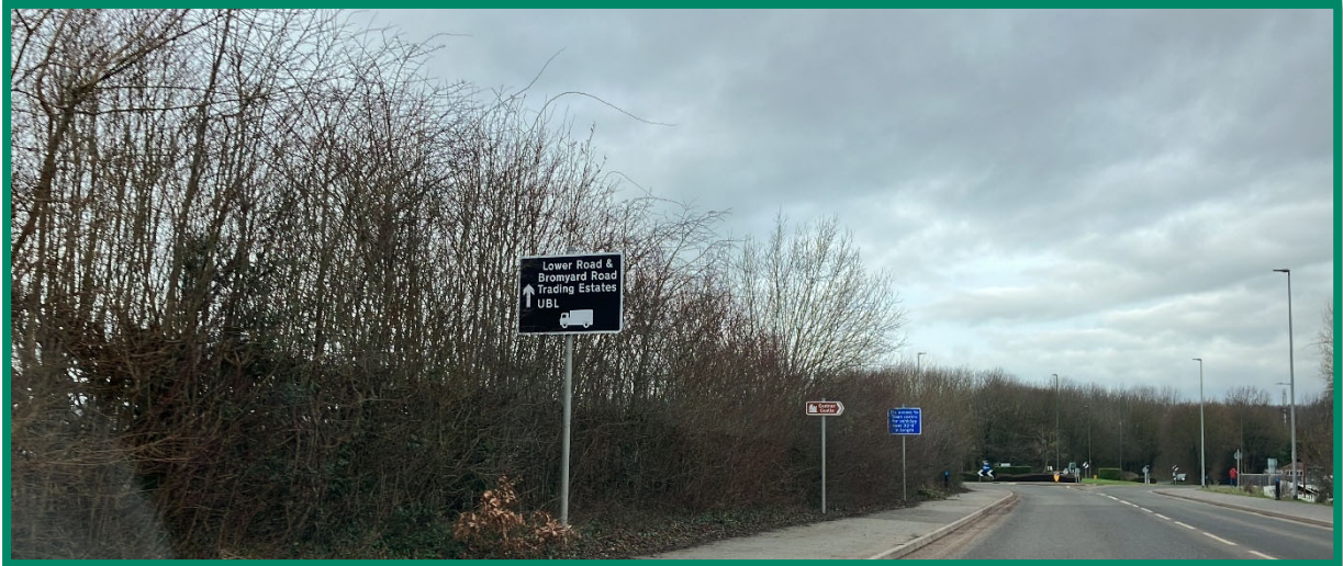
Figure 16 - Existing traffic sign located on the westbound approach to the A449 Leaden Way/ A449 Ross Road roundabout to remain or alternatively subject to sign shown in Figure 16 being retained, this sign is replaced with a new map type sign showing the HGV routes to the industrial areas and weight limit on New Street.
