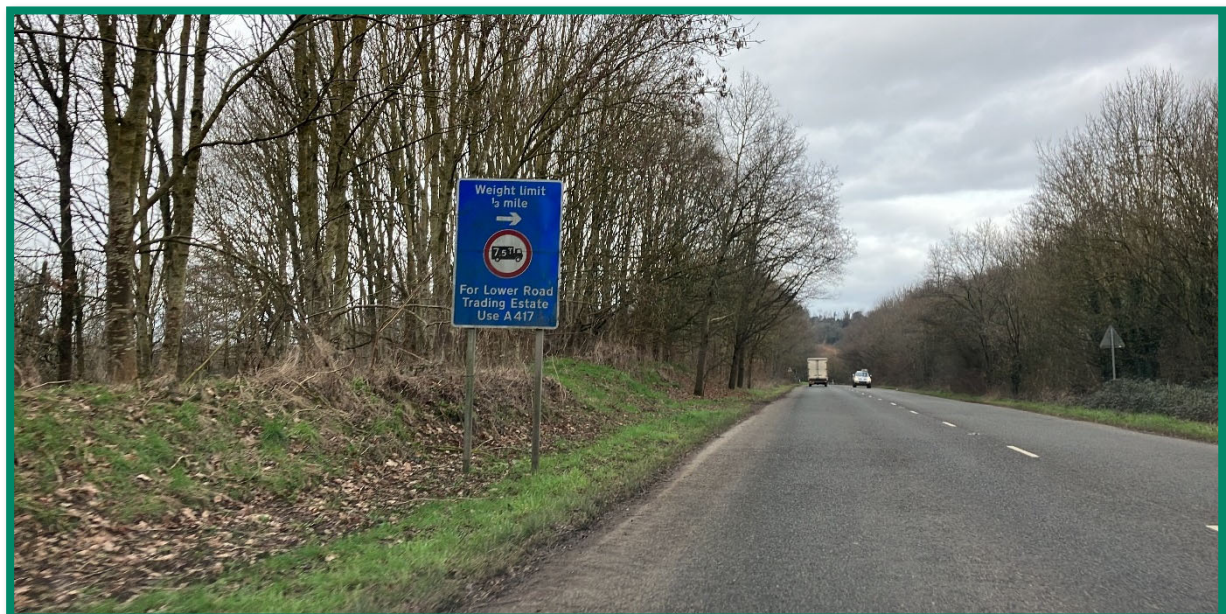
Figure 25 - Existing traffic sign located on the northbound approach to the Leadon Way/Lower Road roundabout. Sign to be replaced if weight limit introduced on Lower Road or as an alternative measure a blue patch could be placed over the '1/3 mile text'.
