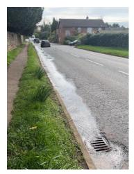
Due to a blocked land drain in private ownership a large volume of water is pouring off the hills onto the footpath and highway in proximity of Ledbury Tennis Club. This issue has been reported multiple times and is resulting in blocked culvert on the highway and splashing of pedestrians and cyclists. I am pushing for action to be taken with the landowner to clear the blockage.
