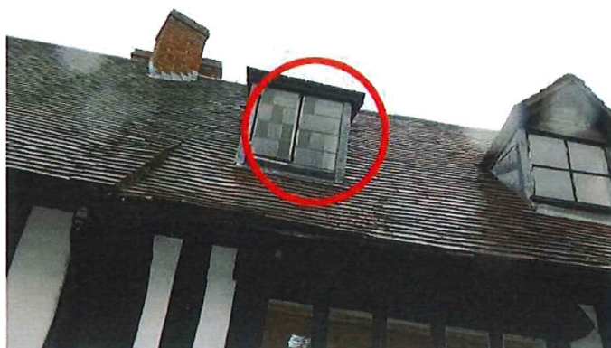
Figure 14 Loose glazing in dormer window circled in red.
