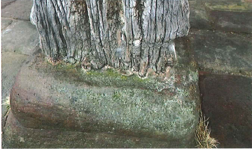
Figure 5. Location C The mortar at the base of the post creates a gutter
