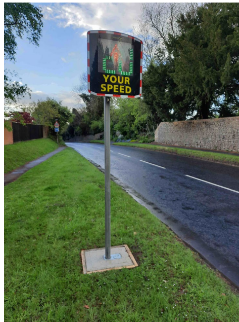
Image showing SID currently installed (May 2021) on the incoming Southend on the approach to John Masefield School
