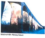
20LED L2102 - Railway Viaduct
