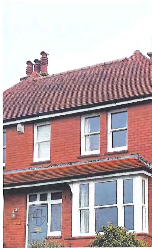
Red/Brown Roof Tiles
