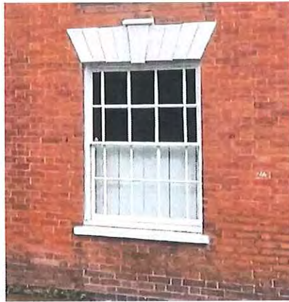
Timber Sash Windows
