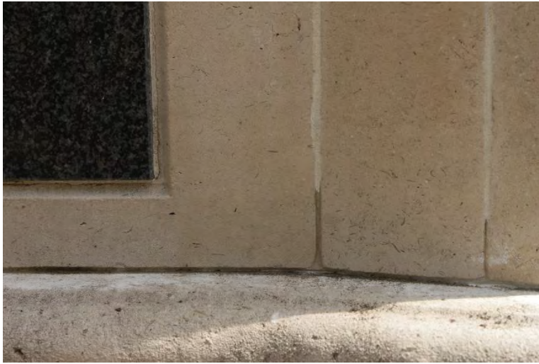
3.1 New pointing to stonework
