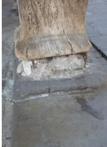
Fig 3.3 Decayed sandstone plinths and steps.
