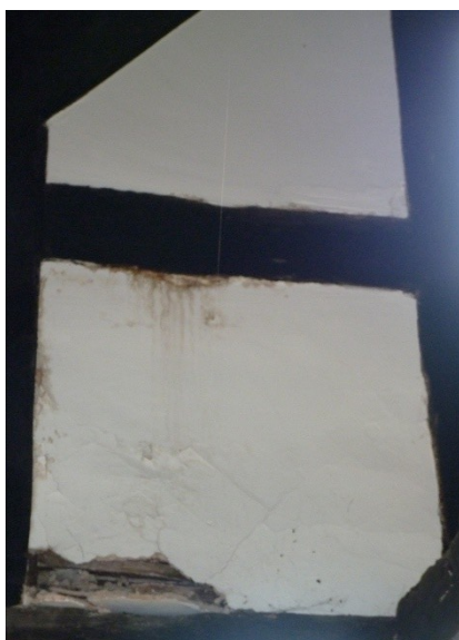
Fig 5.1 Reopened gap at mortice and tenon joint.
