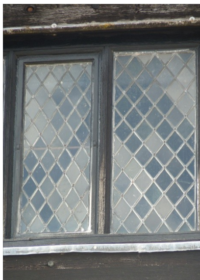
Fig 2.3 Damaged window cill detail. Weathered window frame.
