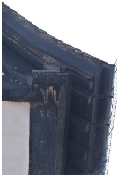
Fig 1.1 Slipped clay plain tile. Old damage to ridge tile.
