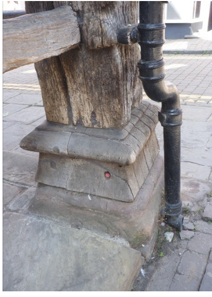
Fig 3.1 Staining and slight decay where rainwater runs back onto timber frame beneath first floor level.
