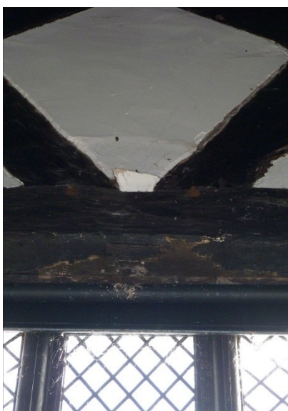
Fig 4.3 Damp staining to sarking board.
