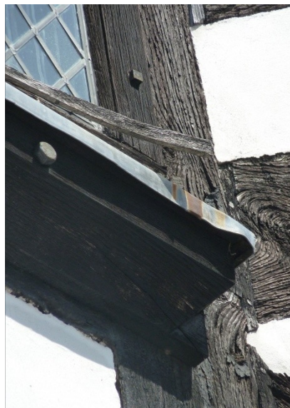
Fig 1.5 Dislodged anti-bird mesh, ongoing decay beneath first floor structure.
