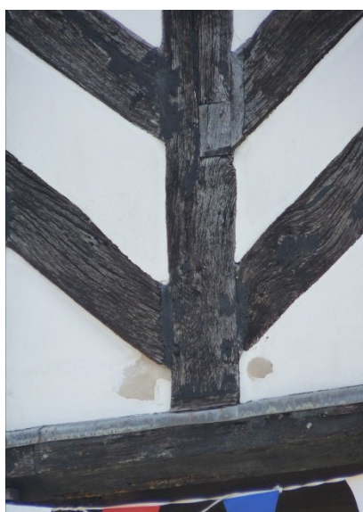
Fig 2.1 Dampness and recent cracks to plaster infill panels.
