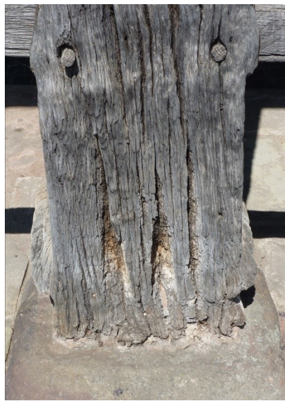
Fig 3.5 Caulking to old shakes in posts falling away.
