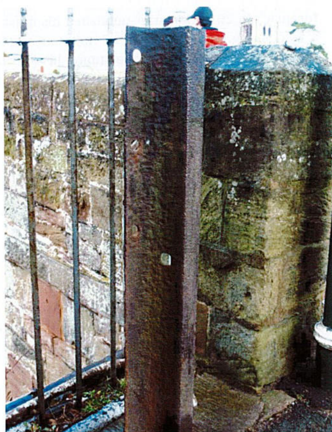
Barlow rail as used on Brunel's broad gauge railway. The rail was spiked to longitudinal timbers with steel tie bars to maintain the gauge. (Hereford old bridge)
