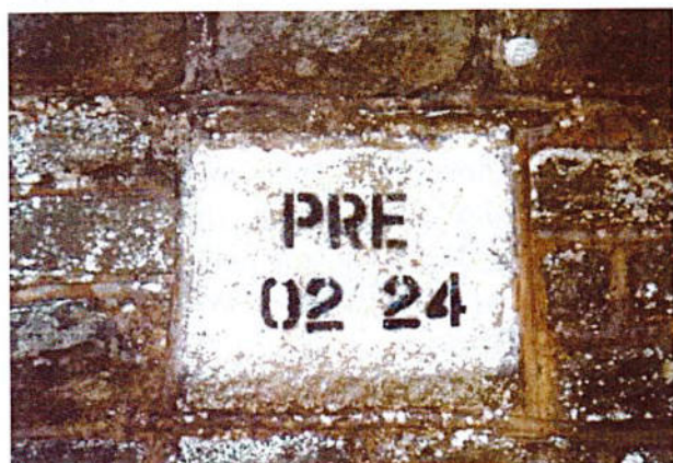
Bridge location and mileage notice (Presteigne branch railway)
