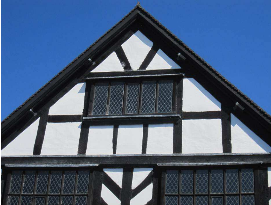
Photo 10 Faded decorations to timber elements to south elevation at high level
