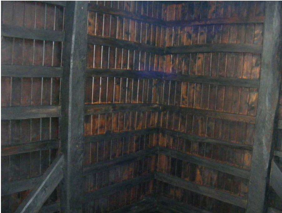
Photo 20 View of exposed timber roof boards forming ceiling and timber joists on roof purlins
