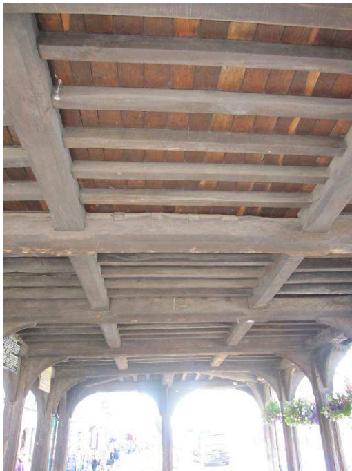
Photo 17 View of underside of first floor showing structural timber framing elements
