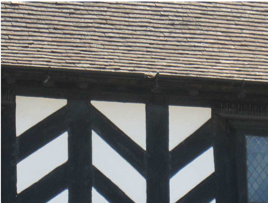
Photo 3 Broken section of guttering to west elevation
