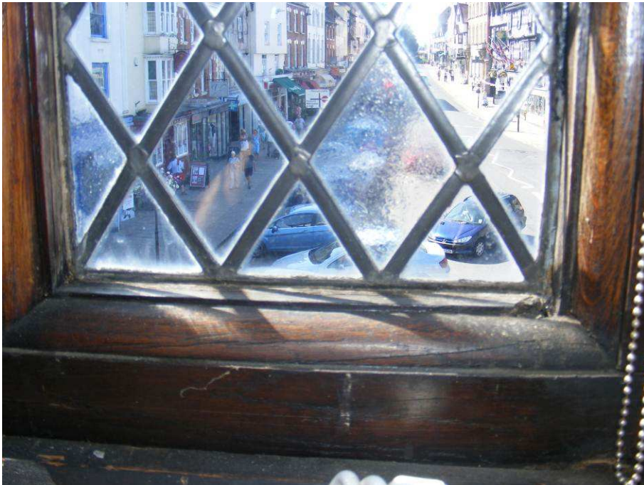
Photo 11 Localised disrepair to base of windows
