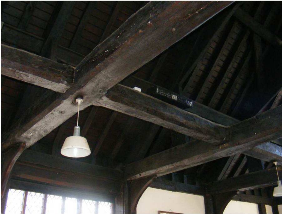
Photo 22 View of fan heaters situated on top of roof beams
