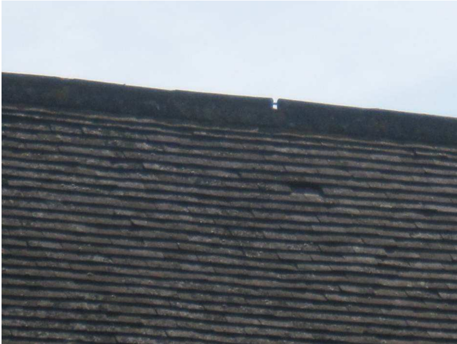
Photo 4 Missing tile and missing pointing to ridge tiles on west elevation
