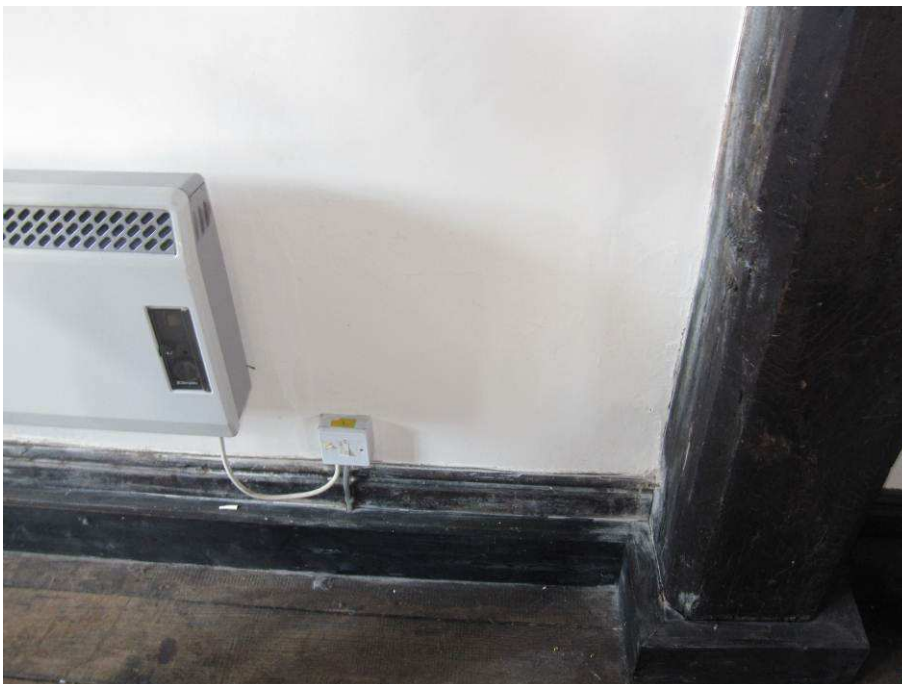
Photo 23 View of night storage heater positioned to perimeter of first floor
