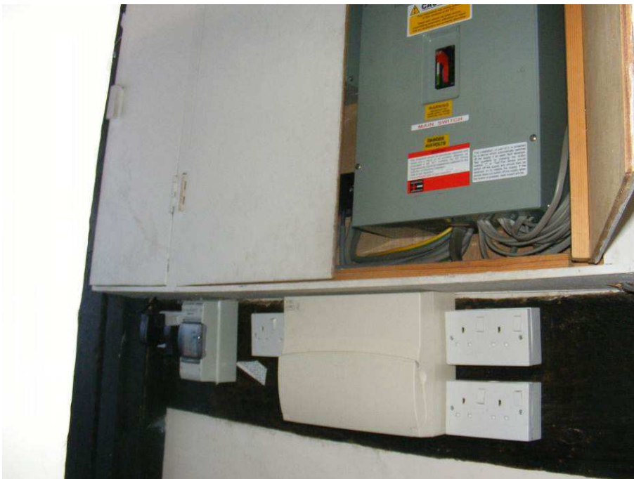
Photo 25 View of mains incoming and isolation switch positioned on north wall
