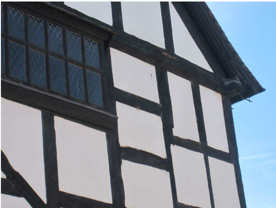
Photo 9 View of high level gable cill to north elevation and 3 no damaged panels
