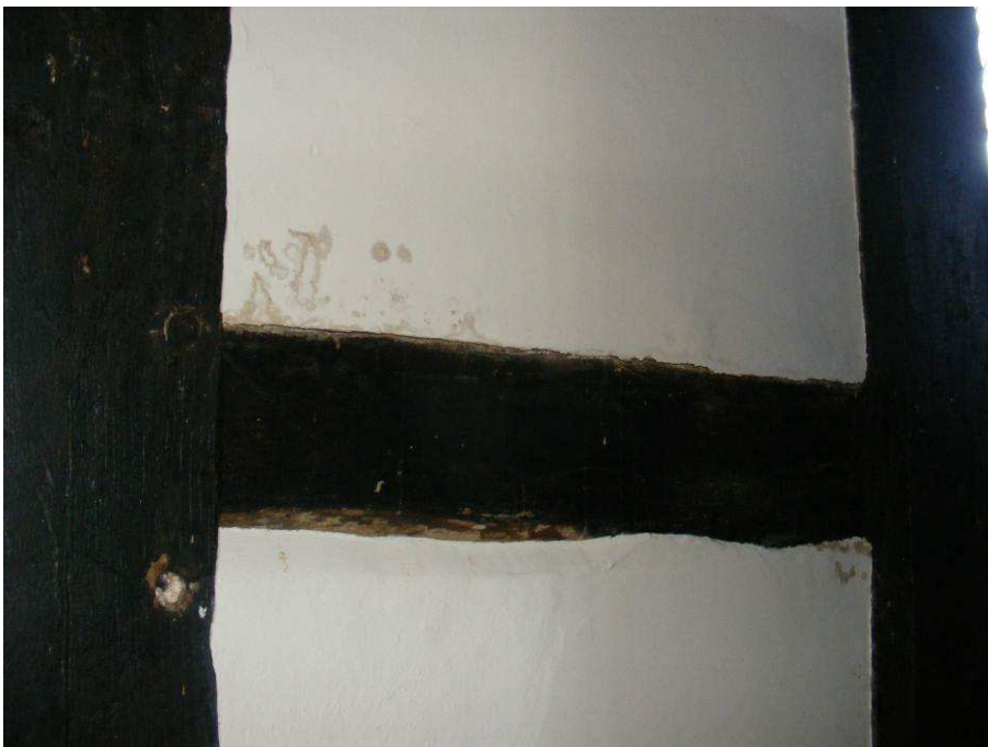
Photo 21 General view of water damage to inside face of infill panel due to defective joints
