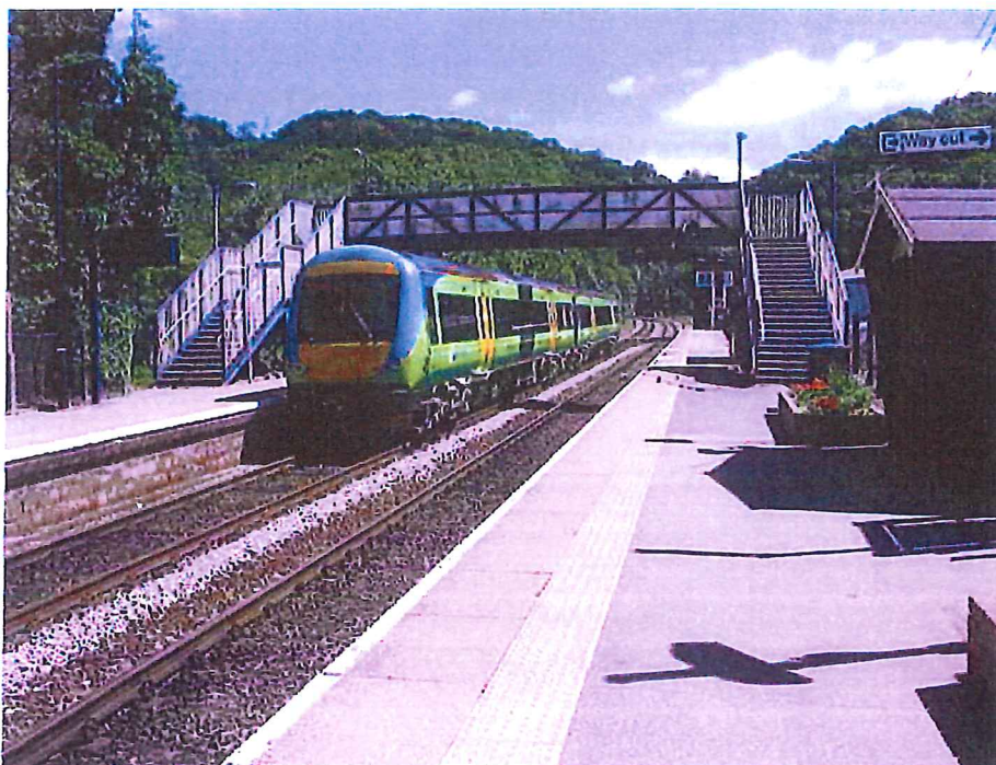
A.3.2 The station as it looks today
