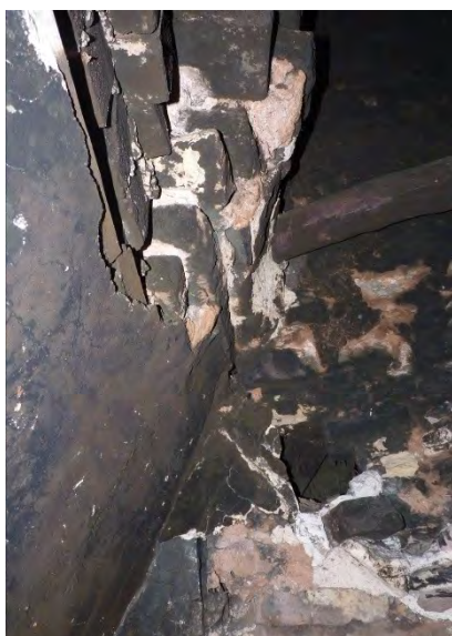
Fig 9.3 Reopened fractures at south west corner of reception.
