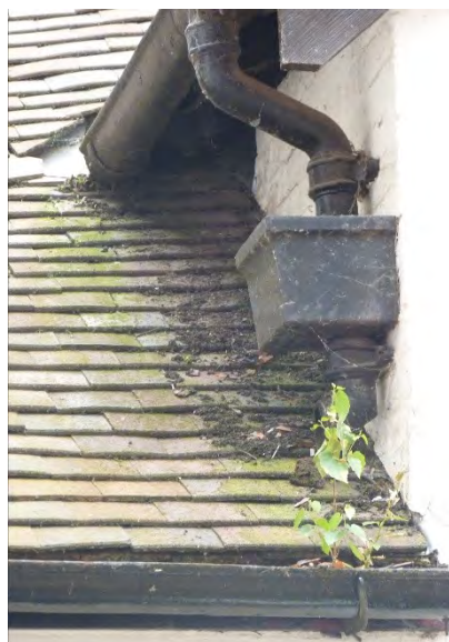
Fig 1.5 Existing lead detailing to north elevation, redirecting rainwater away from roof carpentry.
