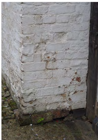
Fig 7.1 Gaps between frame and infill panels to north west corner.
