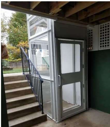
Fig F: Enclosed platform lift, source: assisted-lifting.com
