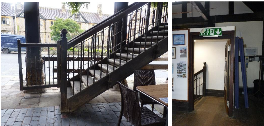
Fig E: Base of Stair and Enclosure at the Top
